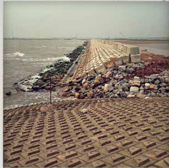
Works on a dike
