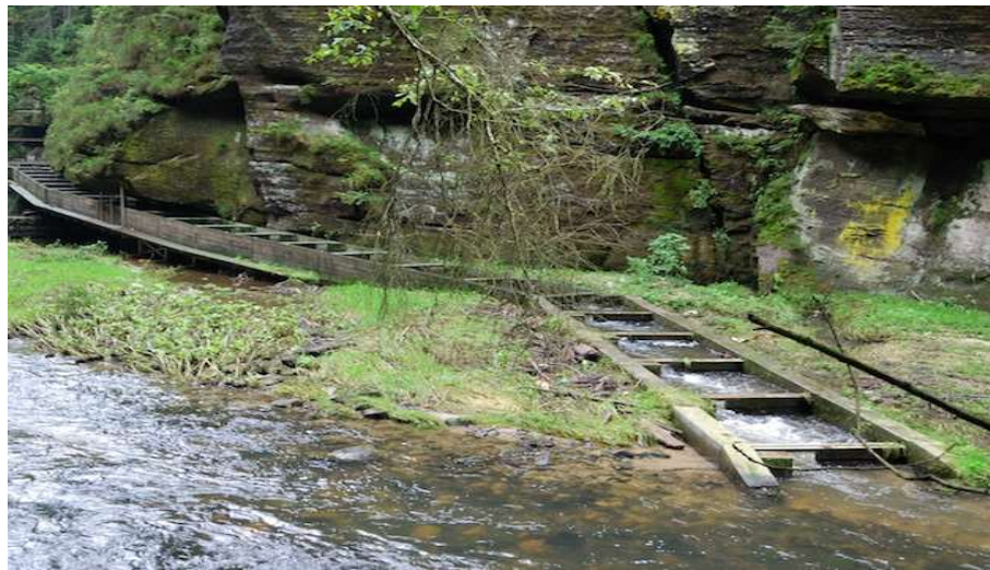
In the Seine-Normandy basin and in the western part of Côte-d'Or, structures have been installed to allow the unhindered passage of fish and sediments. / Source: Hydrauxois
