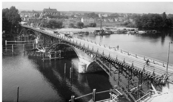
Photograph dating from 1935 showing the works carried out to widen the arches of Pont-de-l'Arche to improve navigation on the Seine
